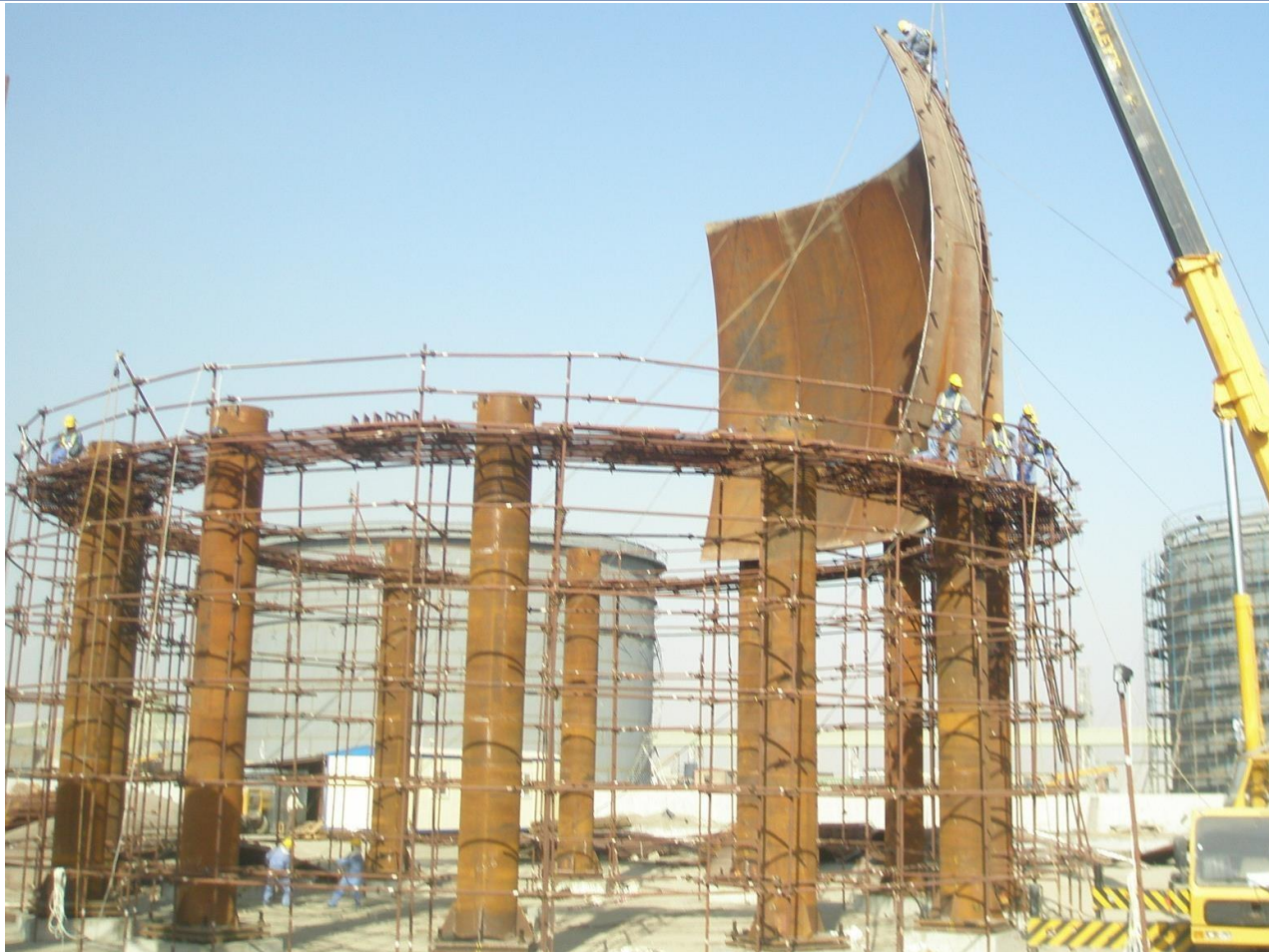
ERECTION OF SPHERE COLUMNS AND EQUATORIAL PETALS
