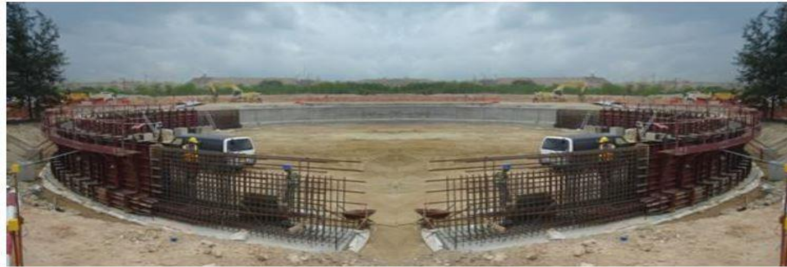
TANK CIVIL FOUNDATION AT SITE (BY LOCAL CIVIL CONTRACTOR)
