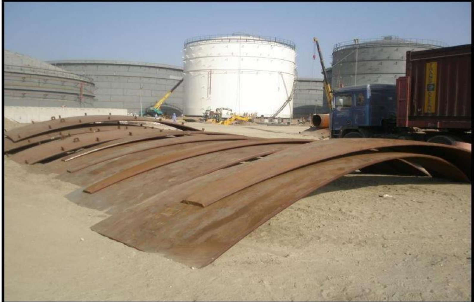
PETROLEUM STORAGE TANK PRE FABRICATED MATERIAL UNLOADING AT SITE
