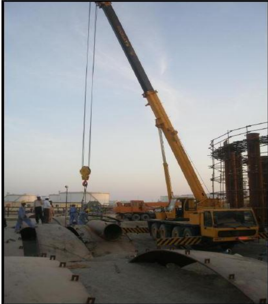
PETROLEUM STORAGE TANK PRE FABRICATED MATERIAL UNLOADING AT SITE
